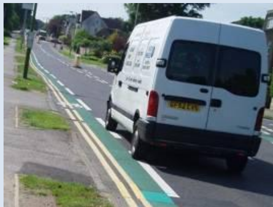
The cycle lanes in North Road are dangerously narrow – less than half the recommended width, exacerbated by traffic islands that push vehicles into the cycle lanes. These are all predictable and unnecessary hazards
